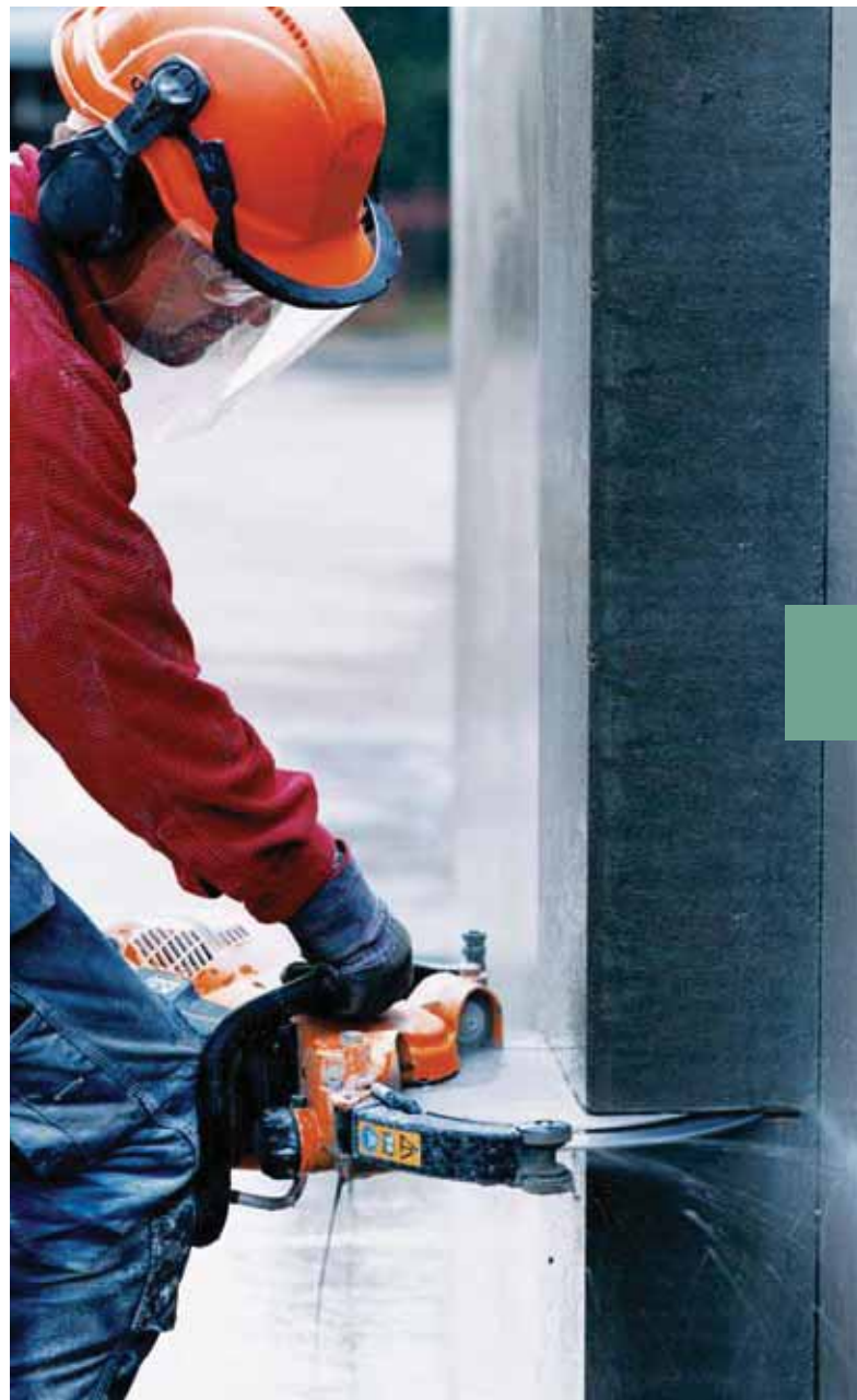
Cutting depth of 10", twice the depth of a traditional power cutter.
