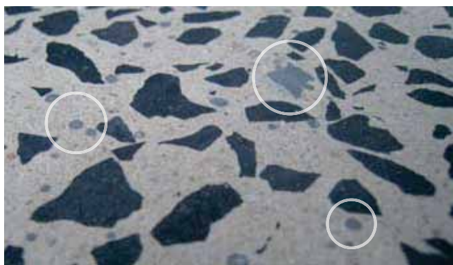
Holes filled when grinding with 120 grit metal-bonded diamonds and GM 3000™.
